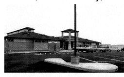
LACO provided engineering, construction materials testing, and Special Inspection services for a new 18,000 square foot building. The project consisted of a multi-story wood frame building with structural steel interior columns and a cast-in-place concrete slab-on-grade founded on continuous and isolated foundations.
