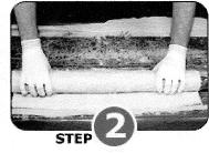
Prepare the resin and wrap the patch around the flow thru packer and secure.
