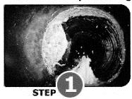
Locate the leak using sewer camera. Clean area to be repaired using rootering or waterjetting.
